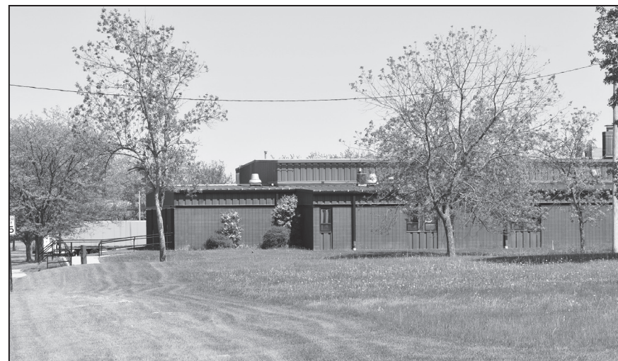
Oconto County hopes to obtain grants to build a new store and training center for the New Beginnings program in this field just west of the New View Center parking lot in Gillett.
