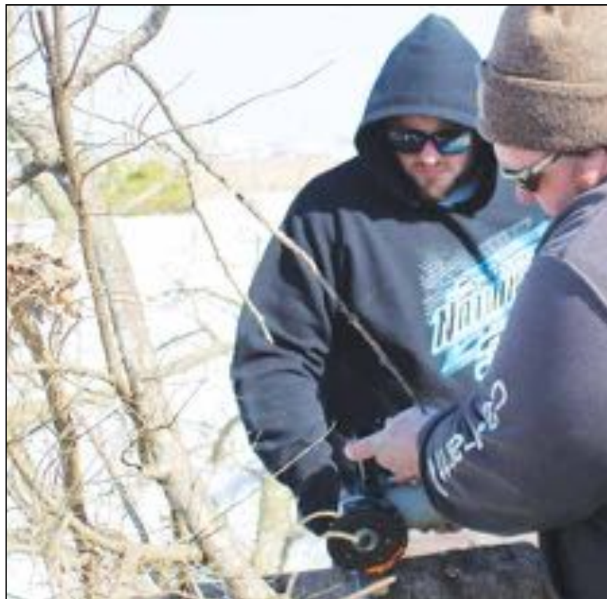
Bobby Smentek, Cecil, right, mans a grinder to cut a piece of cable Feb. 26 while Justin Flaig, Bonduel, holds the cable tight. The pair were among the volunteers building "fish sticks," or fishing habitat structures, on White Clay Lake.
