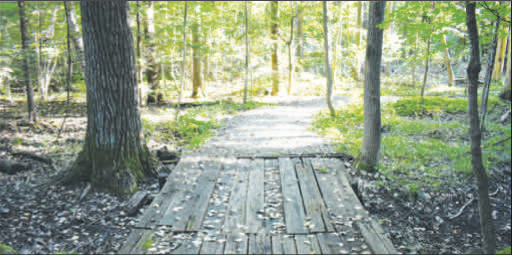
A bridge carries hikers and runners across one of the intermittent streams through the West Side Trail.
