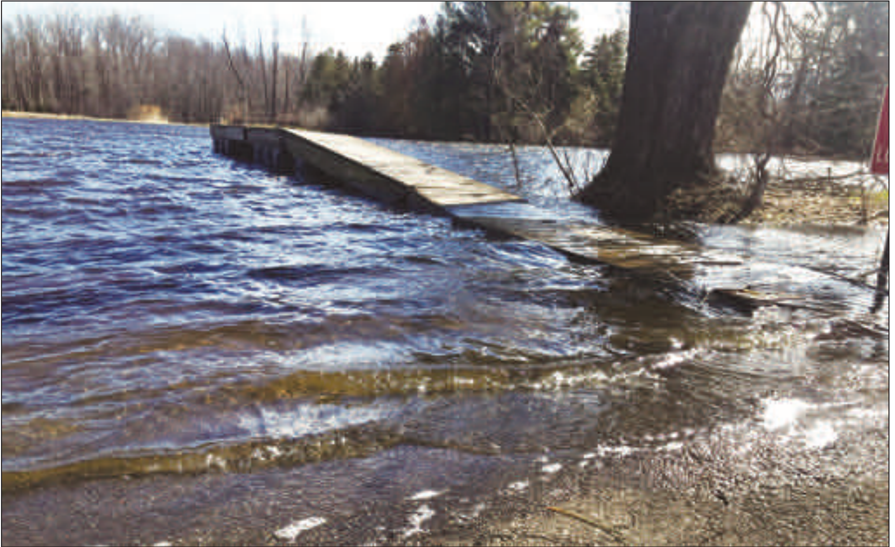
The dock at the Pensaukee Boat Launch is partially submerged April 30, the morning after heavy rain and a strong northeasterly wind caused minor flooding along the bay shore.
