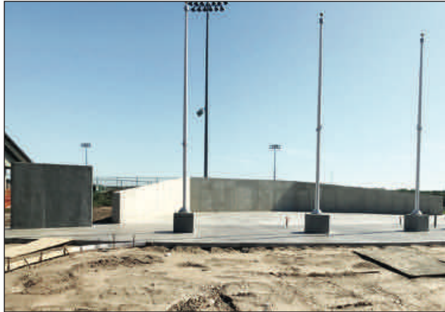
The concrete has been poured, and the Oconto Falls veterans monument is taking shape.
