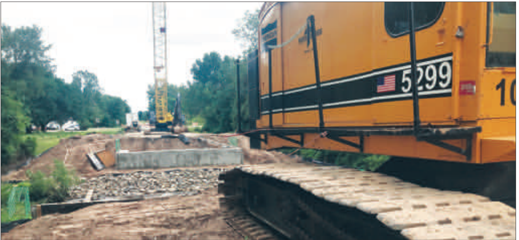
The Pewaukee River bridge on state Highway 32 is being replaced this fall in a project that is expected to detour the road until November.
