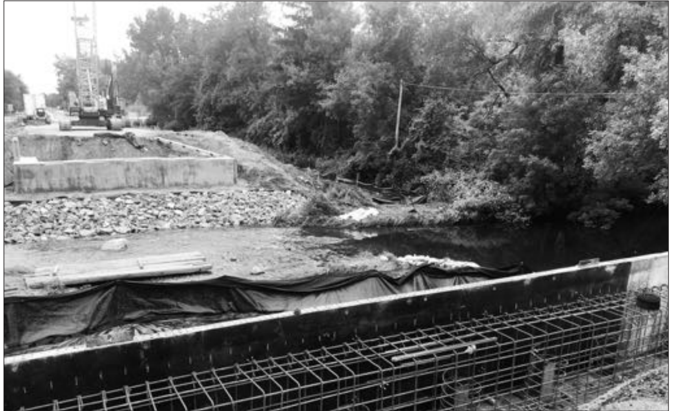
The Pewaukee River bridge on state Highway 32 is being replaced this fall in a project that is expected to detour the road until November.
