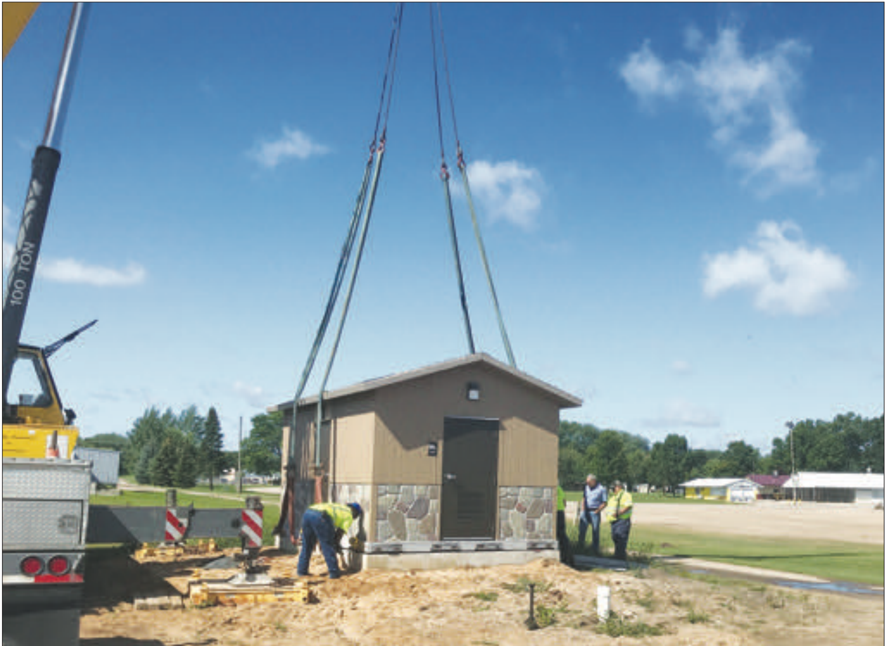
City of Gillett and company workers make the final adjustments after placing the new trailhead serving the Nicolet State Trail at Zippel Park in Gillett on Aug. 27.
