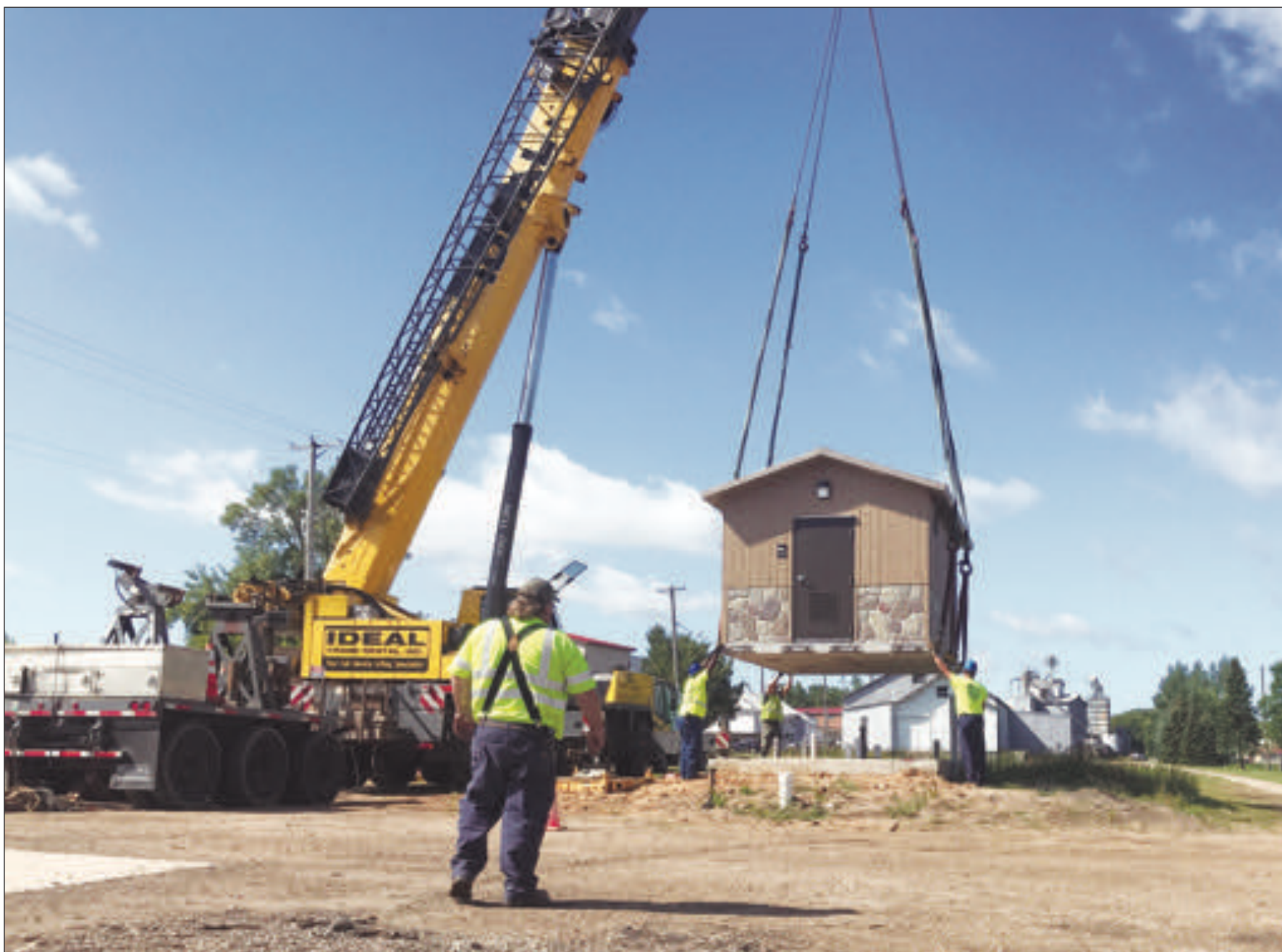
The new building is carefully lifted off the trailer and maneuvered into place.
