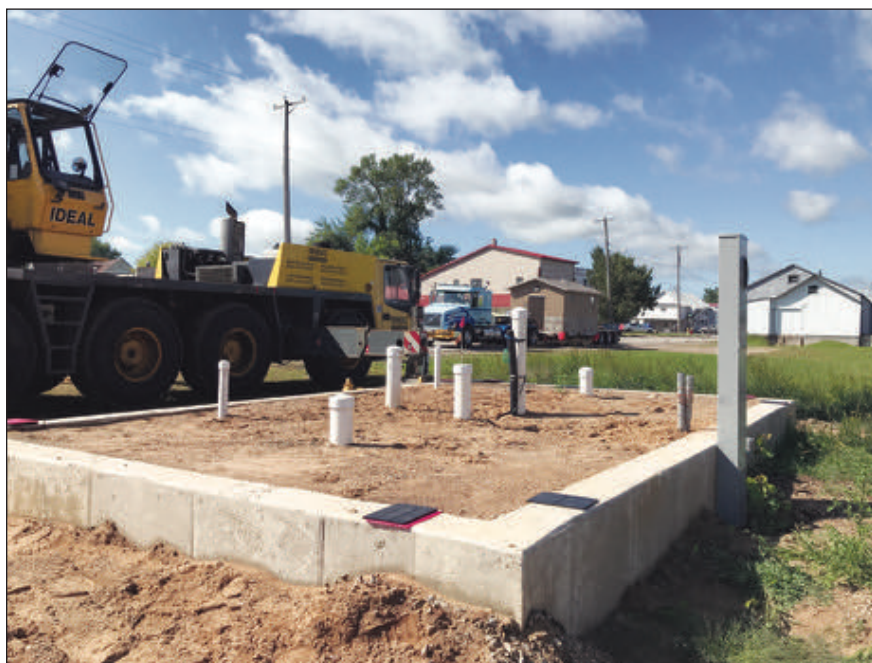
The foundation and plumbing infrastructure was laid weeks earlier.
