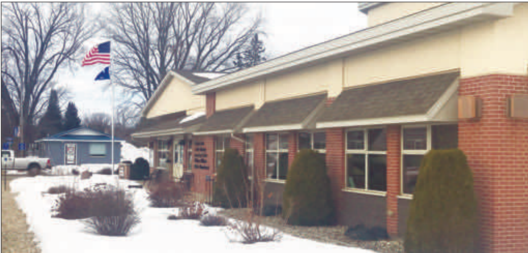
The Suring Municipal Building.
