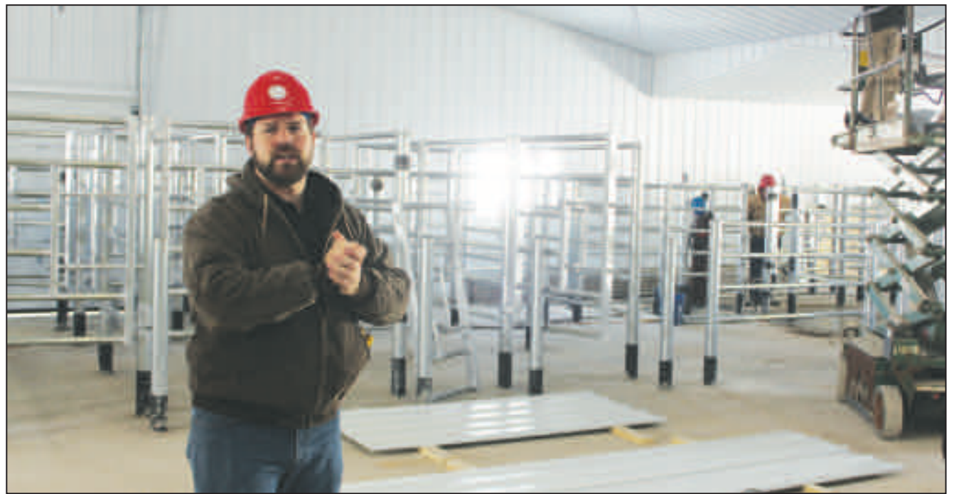
Brian Preder, production site manager for Genex’s Stony Hill facility, stands in front of the partially assembled stalls of the future collection parlor as work crews build in the background. The facility is also expected to get a laboratory to analyze the collections before they’re sent to the processing headquarters in Shawano.
