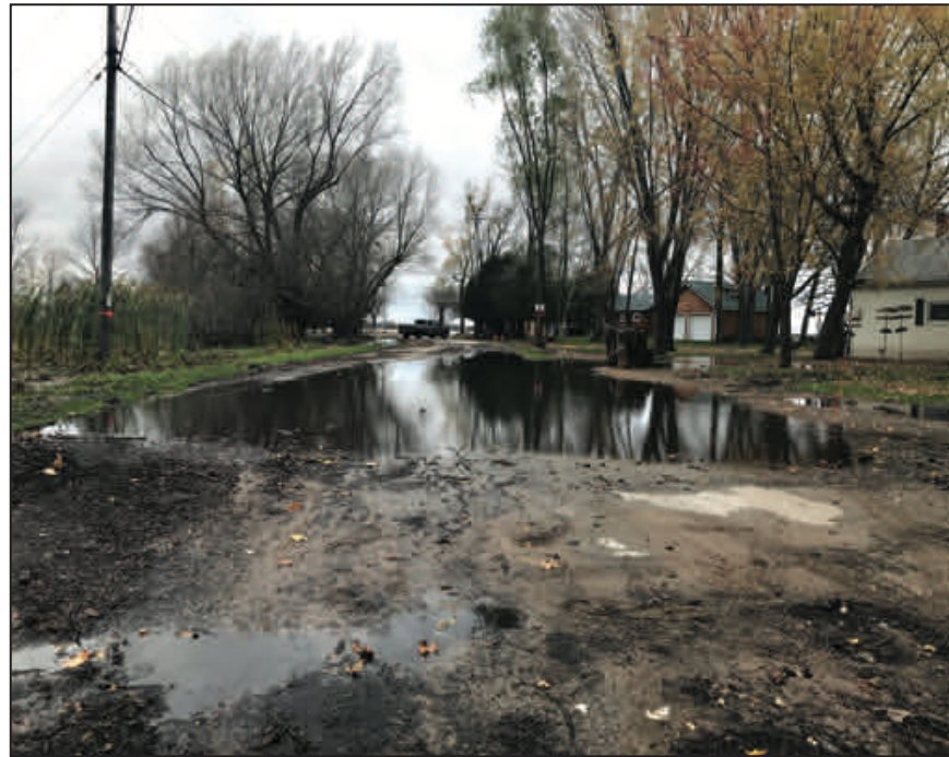
Part of Bayshore Road in the town of Little River washed out in mid-October. The road remains closed to all traffic except residents. Local, state and federal officials are bracing for more flooding as the spring melt combines with record high water levels on the Great Lakes.
