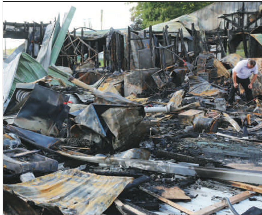
An unidentified inspector looks over the wreckage after an explosion and fire at N4011 Verg Road in the town of Grant that claimed the life of Steve Verg, the owner of the building, and two other victims who succumbed to their injuries in the weeks that followed.
