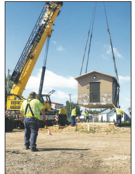
The new trailhead restroom and shower building at the Nicolet State Trail in Gillett is lowered into place. WARREN BLUHM | NEW MEDIA
