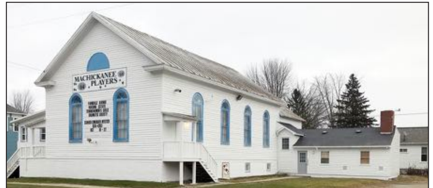
Machickanee plans to use a WPS Foundation grant to raise the foundation under the Park Avenue Playhouse's south wing. WARREN BLUHM | NEW MEDIA
