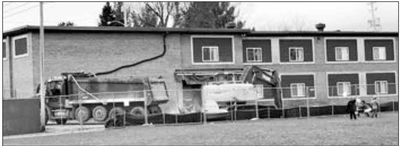
Hanson Sanitation and Excavating prepares the groundwork for the new two-story addition to the Wittenberg Elementary-Middle School as the kids play during recess.
