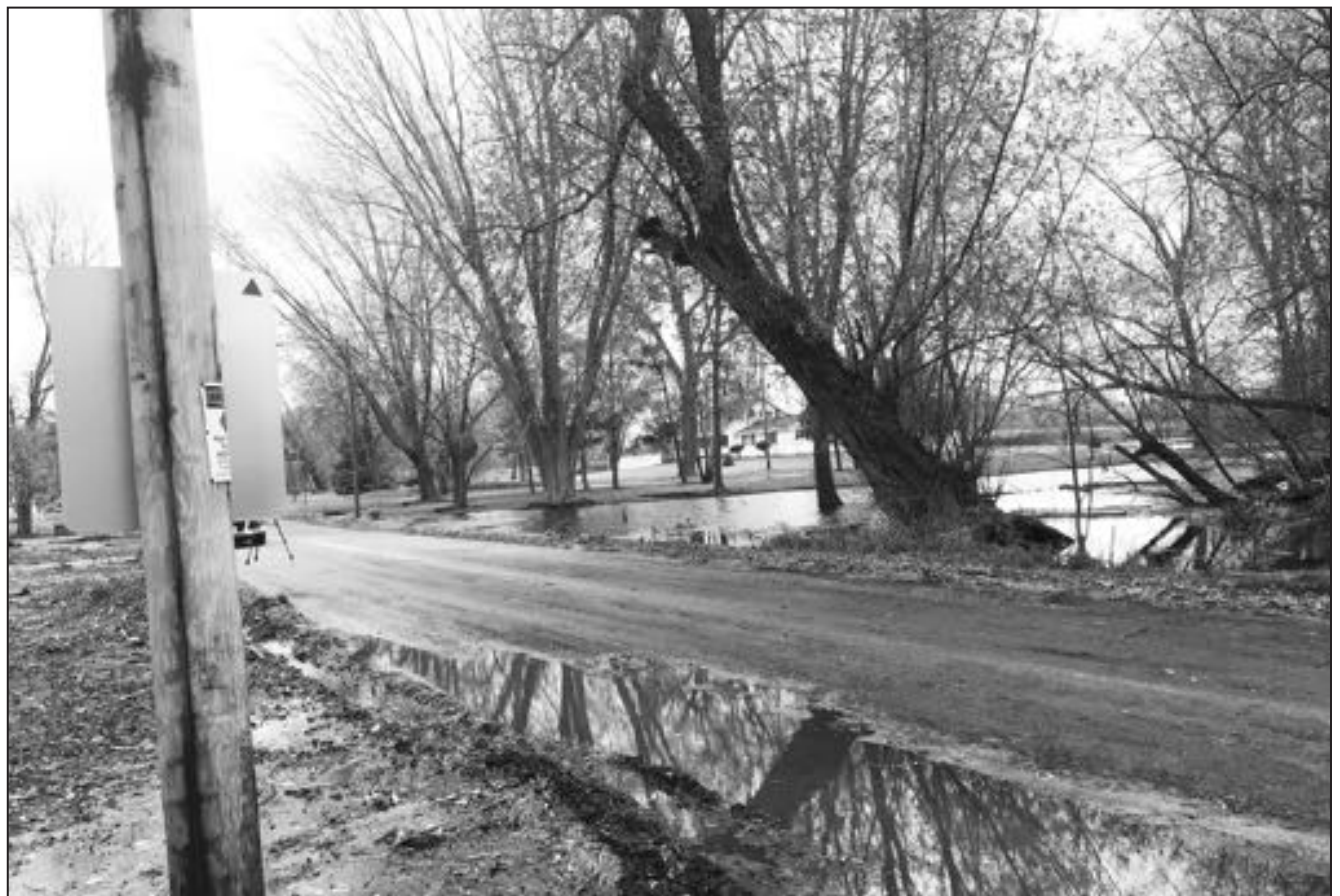
Bay Shore Road was washed out north of Oconto's Breakwater Park after high winds Oct. 15.
