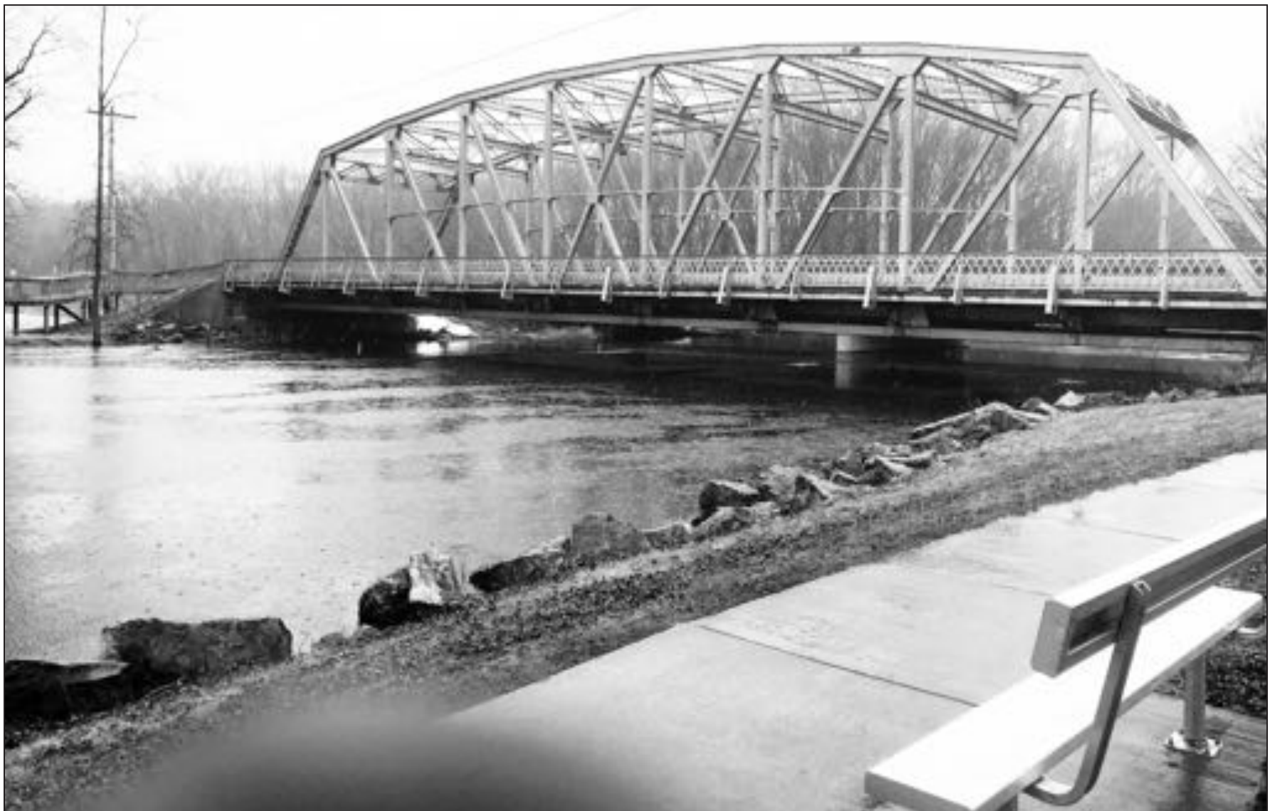
The old bridge in Suring.
