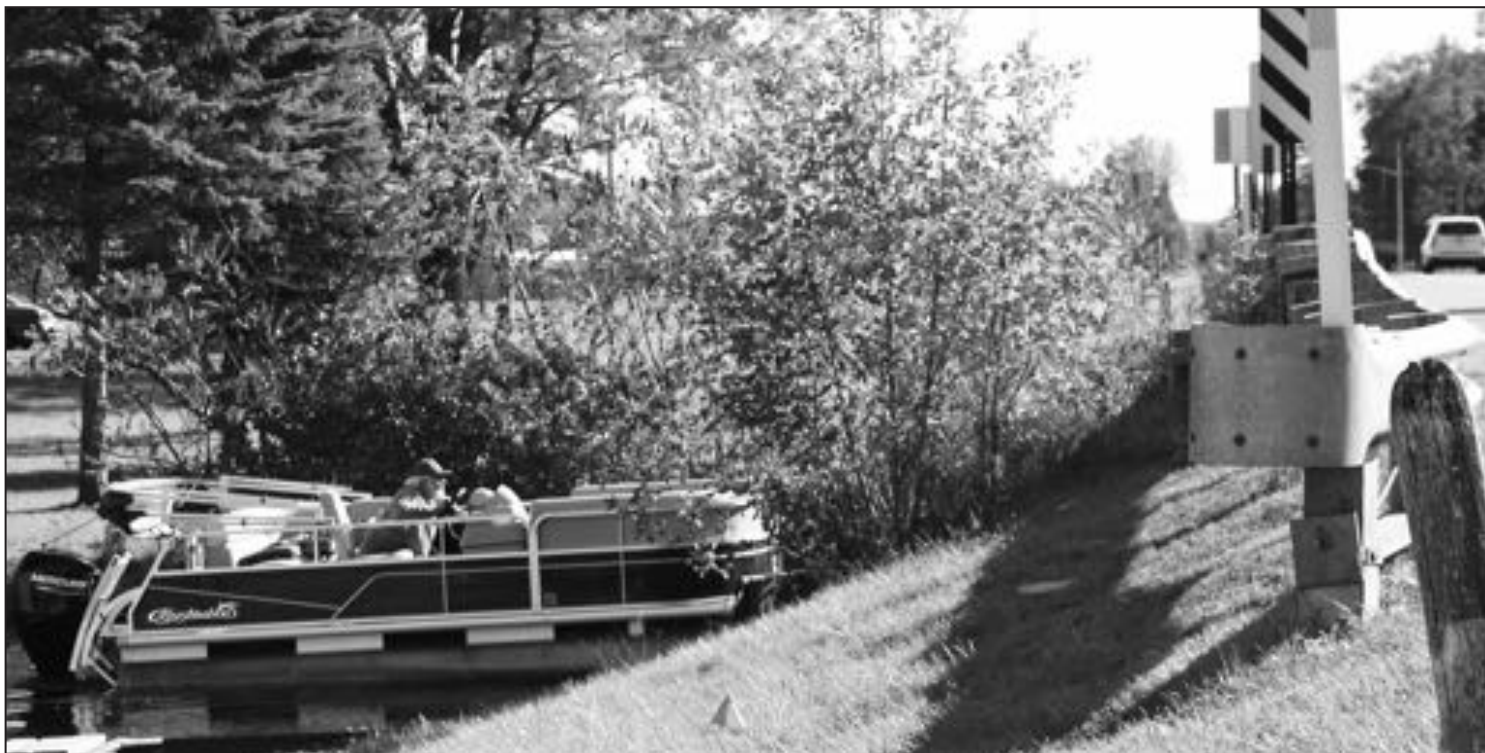
Boaters instinctively duck when approaching the bridge on County Road HHH over what is locally known as The Channel. The bridge is scheduled to be rebuilt. Safety and access concerns surfaced at a public information meeting Wednesday as bridge improvement options were outlined.
