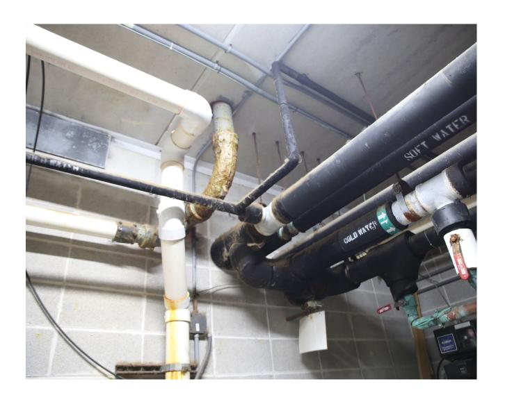
Several rusted cast-iron pipes have swollen to be much larger than they were originally and are considerably weakened. Should the pipes burst, water from the pool would flood the mechanical area.
